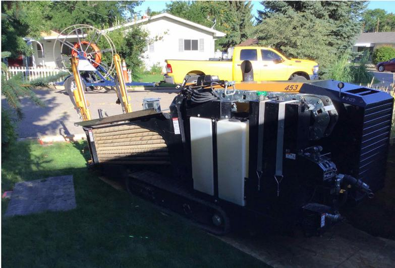
Boring Machine and Conduit
