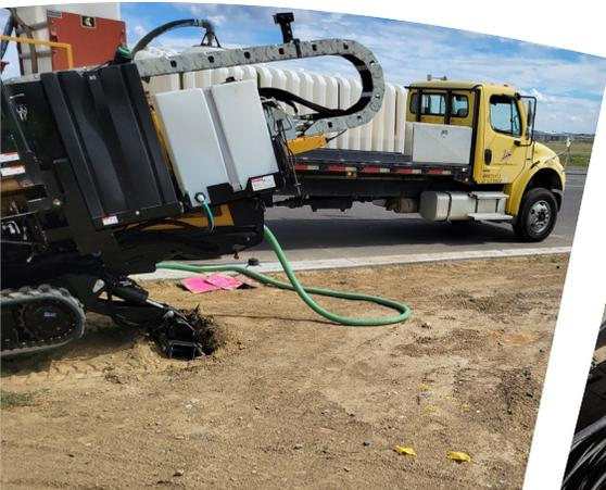
Bore Machine and Water Truck
