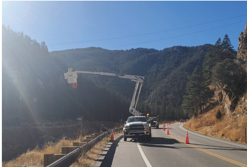
Aerial Fiber Installation
