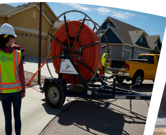
Pulse Staff Overseeing Conduit Installation
