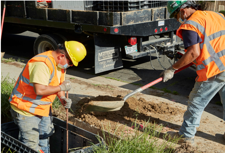
Handhole Installation
