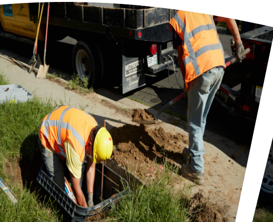
Fiber and Vault Installation
