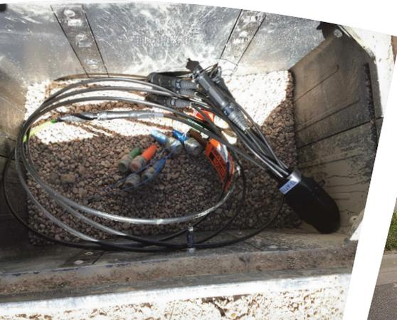
Fiber Access Terminal for Premise Fiber Installation
