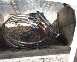
Fiber Access Terminal for Premise Fiber Installation
