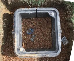
Hand Hole Hydro Excavation and Installation Before Backfill
