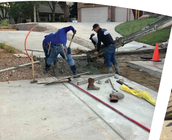
Placing Concrete
